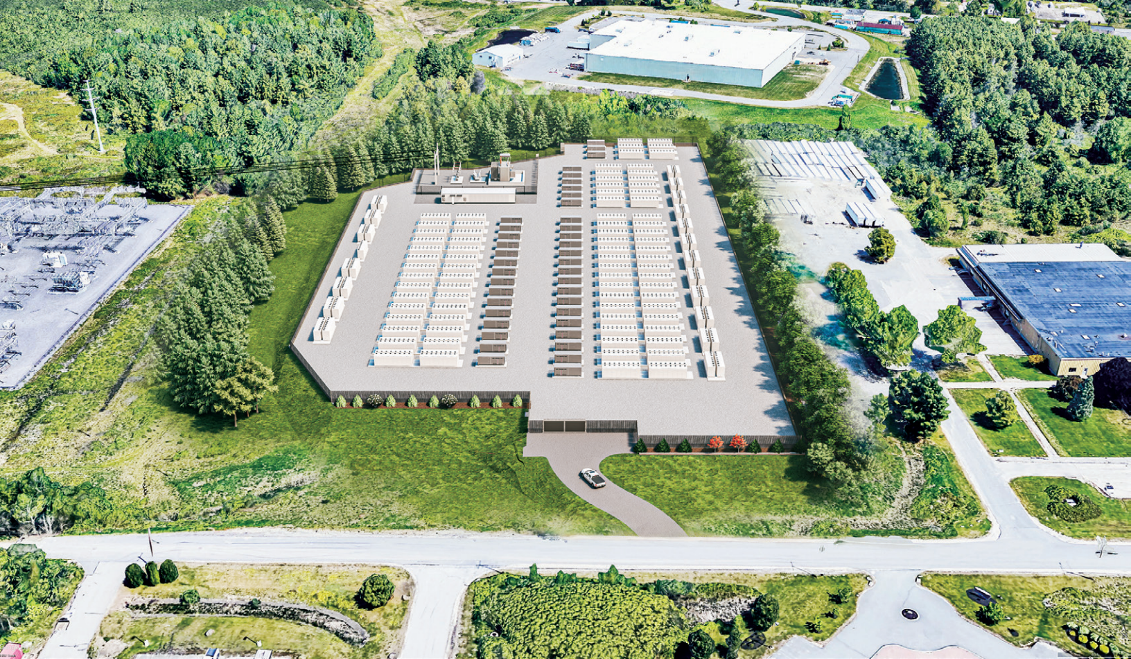
The soon-to-be started Cross Town Energy Storage Project will be a 175 MW/350 MWh battery storage project located in the town of Gorham, Maine. Artist Rendering courtesy of Plus Power.
