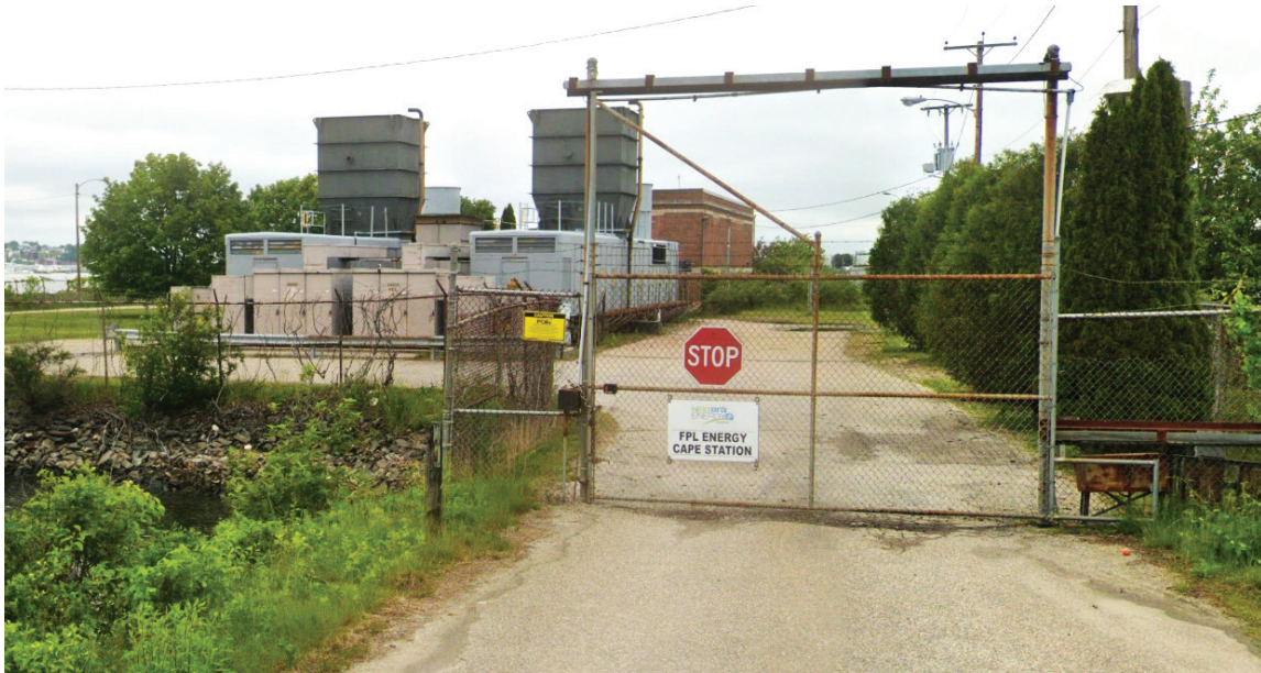
The Cape Gas Turbine in South Portland was built in 1970 as a simple cycle gas-turbine facility, with a capacity of 35 MW. Photo: Image Capture, June 2019, © 2024 Google.
