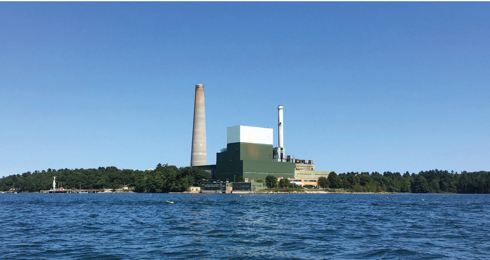
Wyman Power Station is an oil-fired peaker power plant in Yarmouth, Maine.
