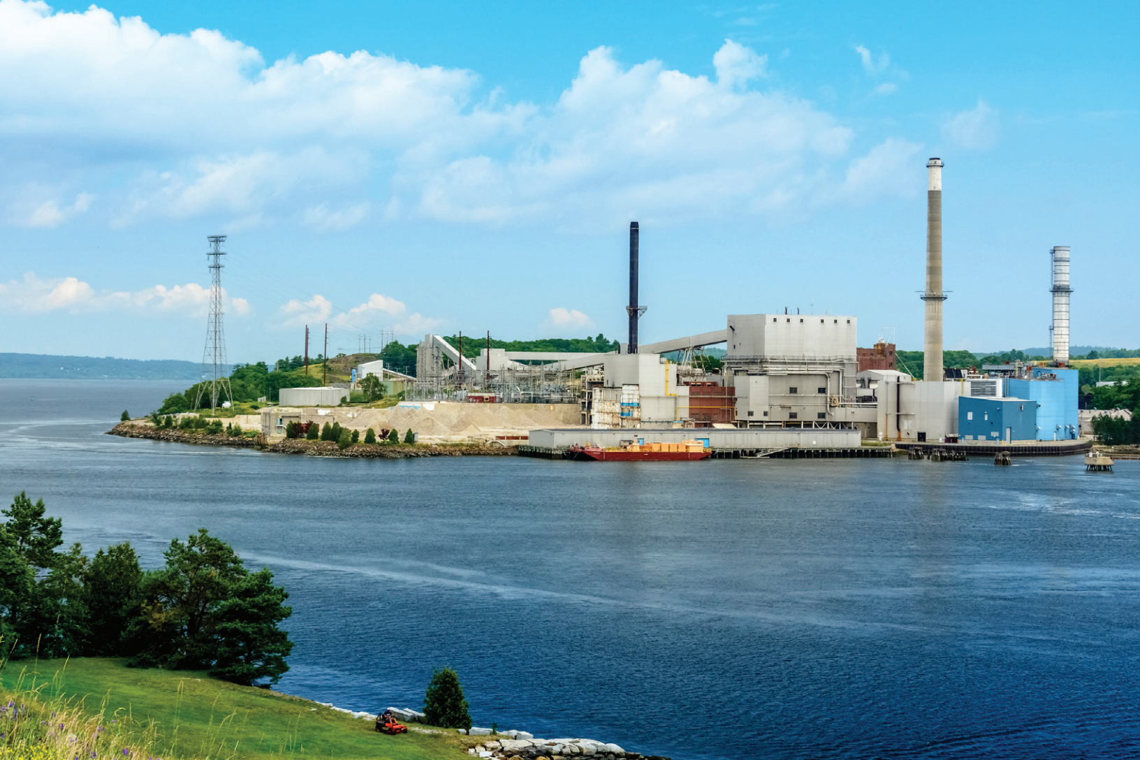
The Bucksport Generation Power Station is a gas-fired peaker power plant at the site of the former Verso Paper Mill in Bucksport, Maine. Photo gkenmo/iStock
