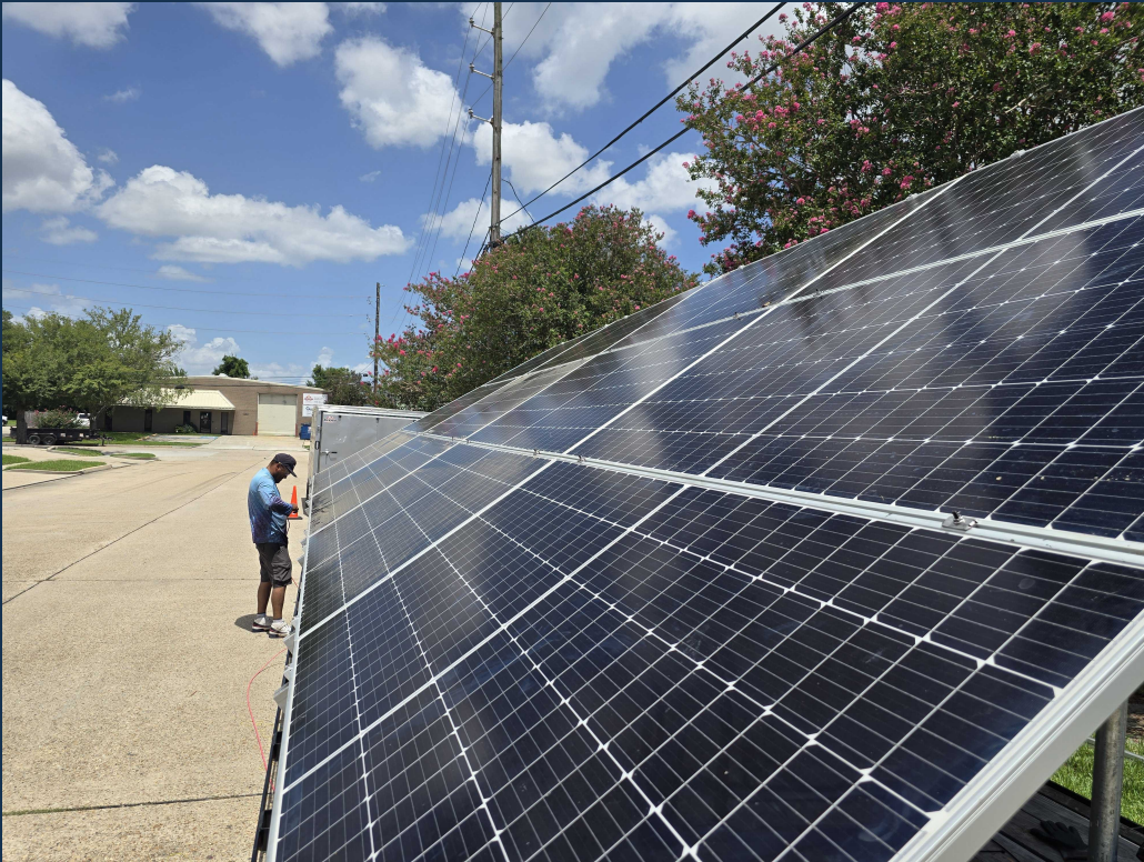
Building the array
