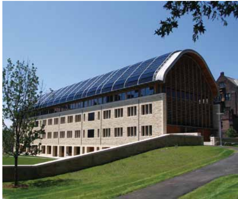
Solar panels on the roof of Kroon Hall, Yale School of Forestry & Environmental Studies, New Haven, CT
