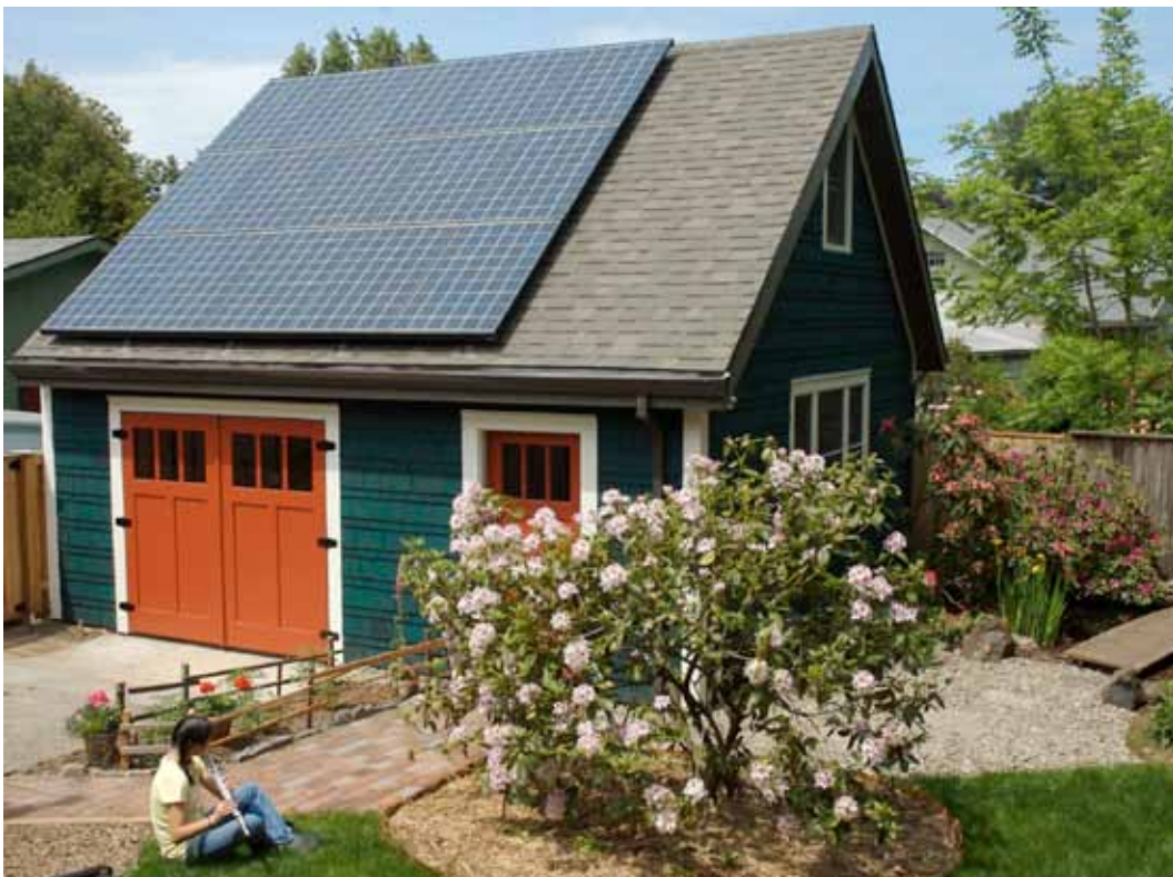
Residential PV project supported by the Energy Trust of Oregon
