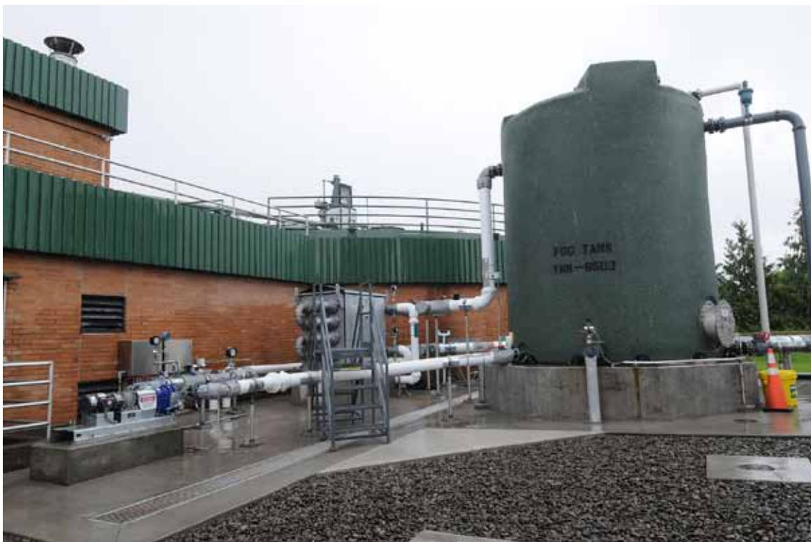
The City of Gresham Wastewater Treatment Plant. By collecting and diverting fats, oils, and grease (FOG) out of the wastewater collection stream and using anaerobic digesters to create biogas from the waste, this system enables the wastewater treatment facility to reach its net-zero energy use goals.
