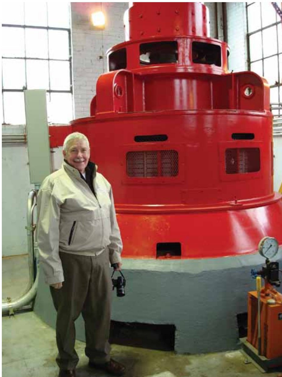
Energy Trust's board president John Reynolds attended the ribbon-cutting for the city of Albany's 500 kW hydro project. The turbine and generator are part of the city's drinking water system.
