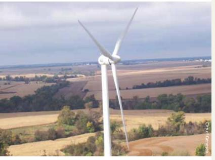
The City of Geneseo recently installed two Vensys 77 1.5 MW gearless turbines that will provide roughly 12% of the electricity consumed in Geneseo.
