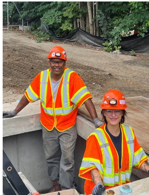
Utility pipefitters on the job in Framingham, Massachusetts. Credit: Eversource Energy.
