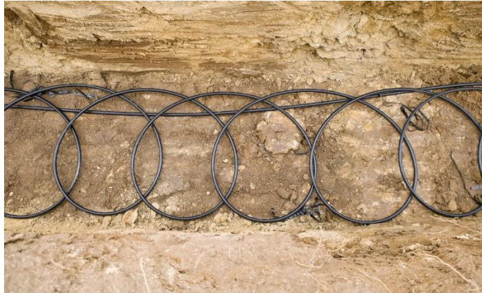
Geothermal pipe coils at the bottom of a trench. Credit: BanksPhotos/iStock.
