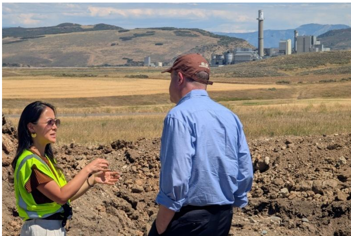
Bedrock Energy CEO Joselyn Lai, wearing a safety vest, gestures while explaining thermal energy network design to Colorado Governor Jared Polis. They stand beside an earthen trench at the construction site of the Town of Hayden Northwest Colorado Business Park Geothermal Project, with the Hayden Coal-Fired Power Plant and rolling hills in the background. Credit: Bryce Carter, Colorado Energy Office.
