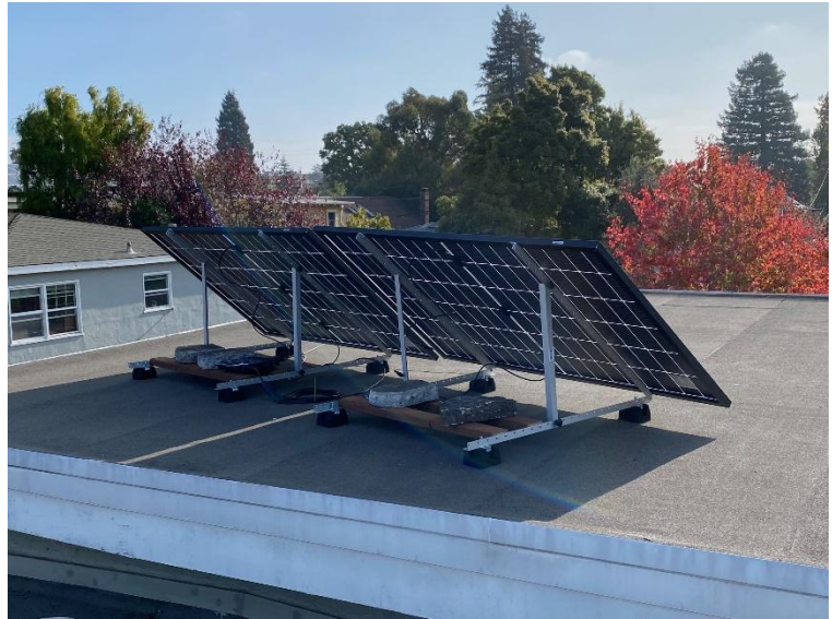
Plug-in solar system installed on a rooftop in Berkeley, CA. Photo Credit: CESA.
