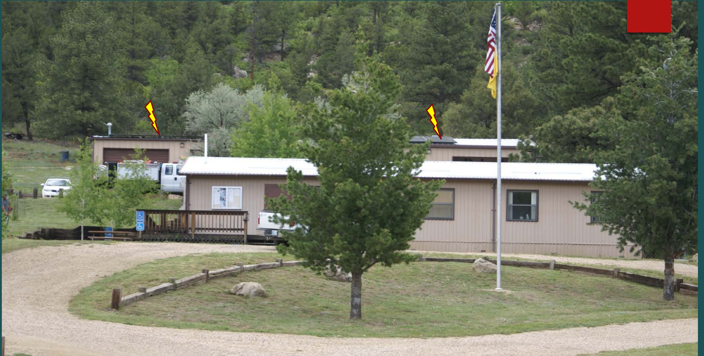
Cimarron Forestry District Office from US 64 road with solar panels installed.
