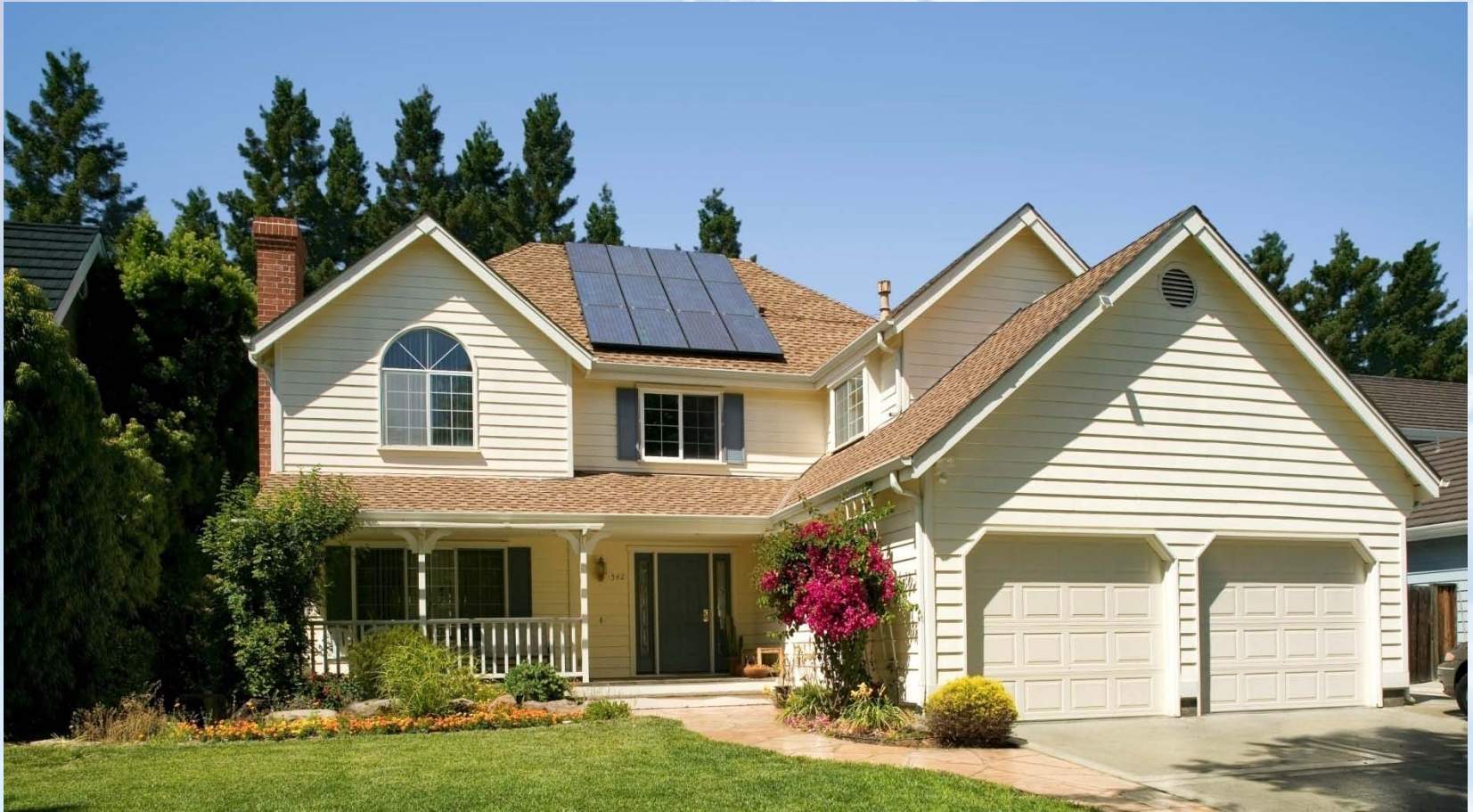
Residential PV System Photo Courtesy of SolarCity.
