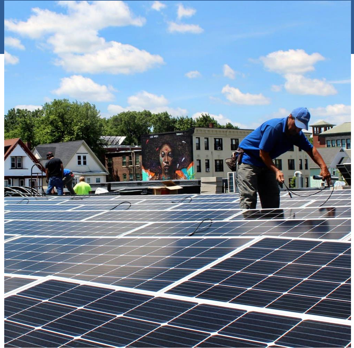
Rooftop solar installation in Dorchester, MA. Credit: Resonant Energy
