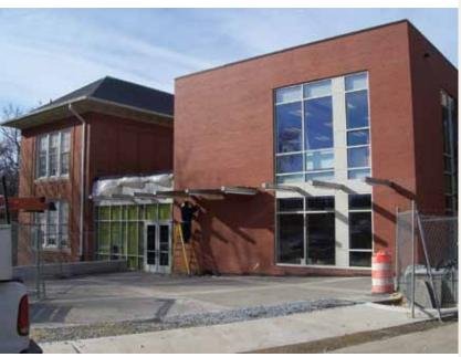
TRF Energy financed the energy retrofit of existing space and an energy-efficient addition at the Latin American Montessori Bilingual Public Charter School in Washington, D.C. The energy measures included a high-efficiency modular boiler heating system, a high-performance building envelope with daylighting features, energy-efficient lighting fixtures and controls, and a green roof for capturing storm water.
